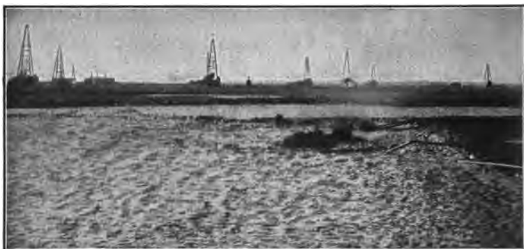
FIG. 108.—Oil well, derricks and pipes discharging crude petroleum into a pool containing many thousand barrels, Muskogee, Okla. (Standard Oil Co.) This wasteful method is often necessary where every land owner works wildly to dig wells on his land, and the wells gush (20,000 to 60,000 barrels per day), so much that even pipes cannot carry it away.
